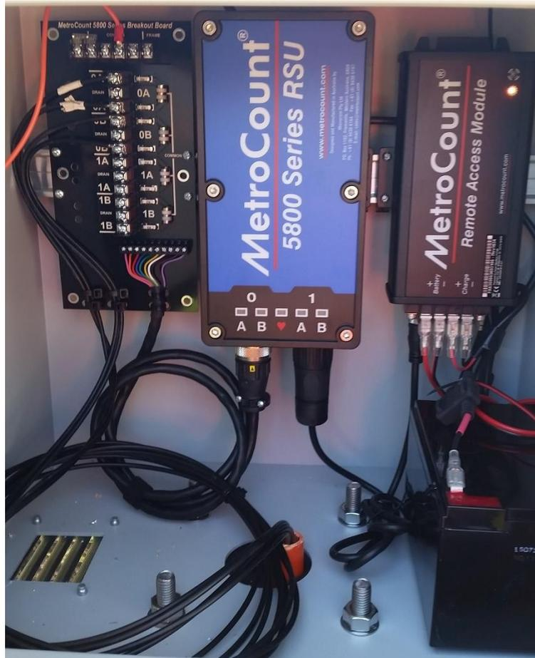
**Figure 5 - Cabinet internals showing connections**
