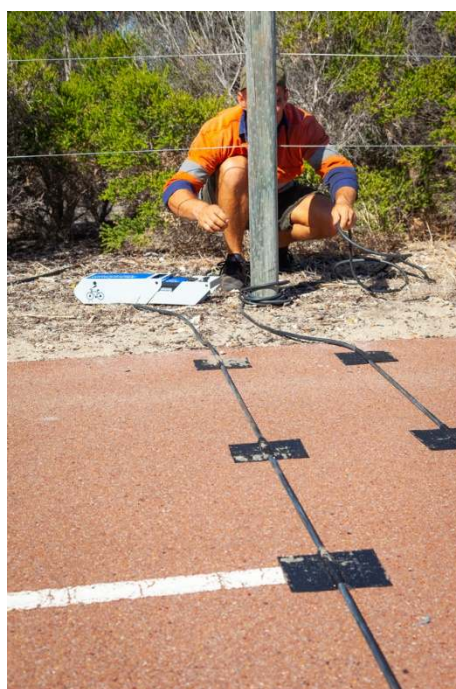
Pic 4. above: Using strips of Bitumen Tape across the length of the tubes to secure the tubes to the Bike path surface
